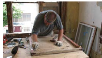
Careful repair of original wood windows can extend their life indefinitely.
